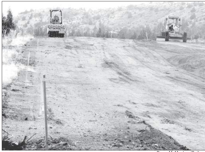
Preliminary work includes new roadways.
