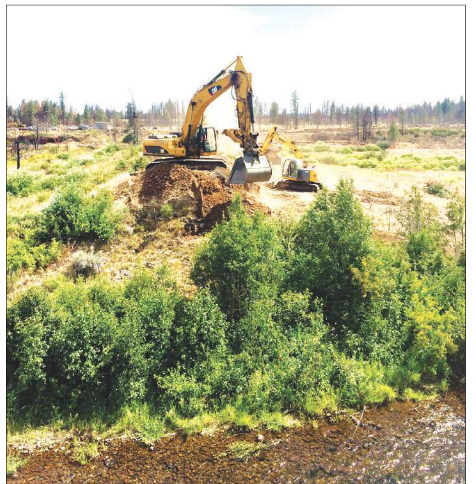
Removing the lower berm
