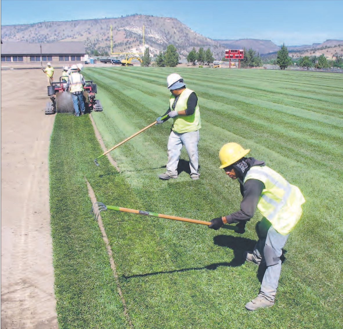
Cedar Landscape crew rolls out the sod on the academy football field.
