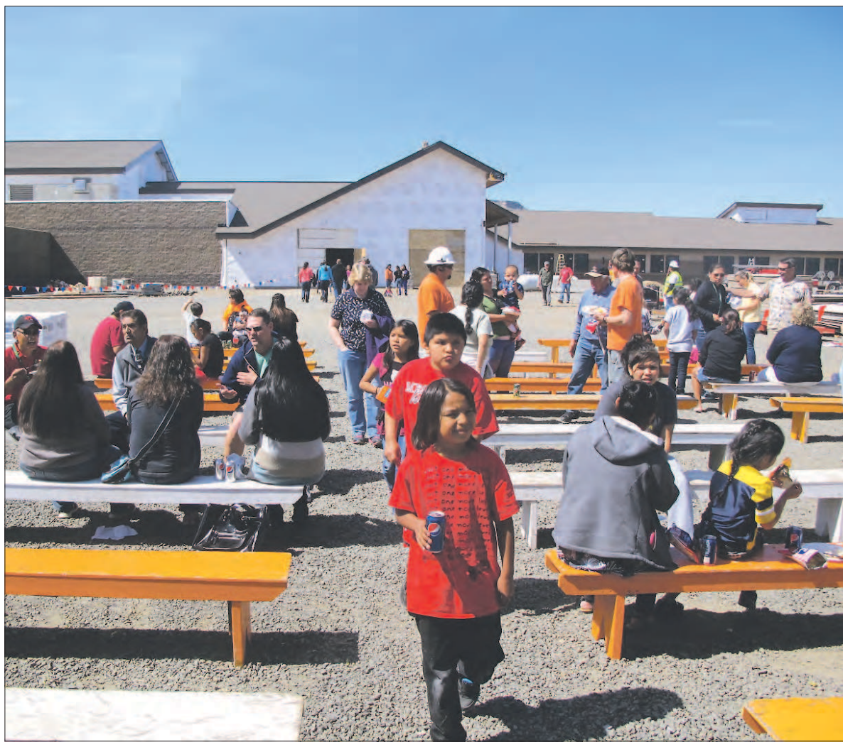
Students and other community members visited the K-8 Academy last week during the open house. The commons area is the tall structure in the center; the k-2 wing is the right, and the gymnasium is tall structure to the left.
