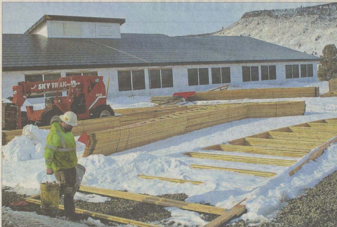
Construction continued through the recent snowy weather.
