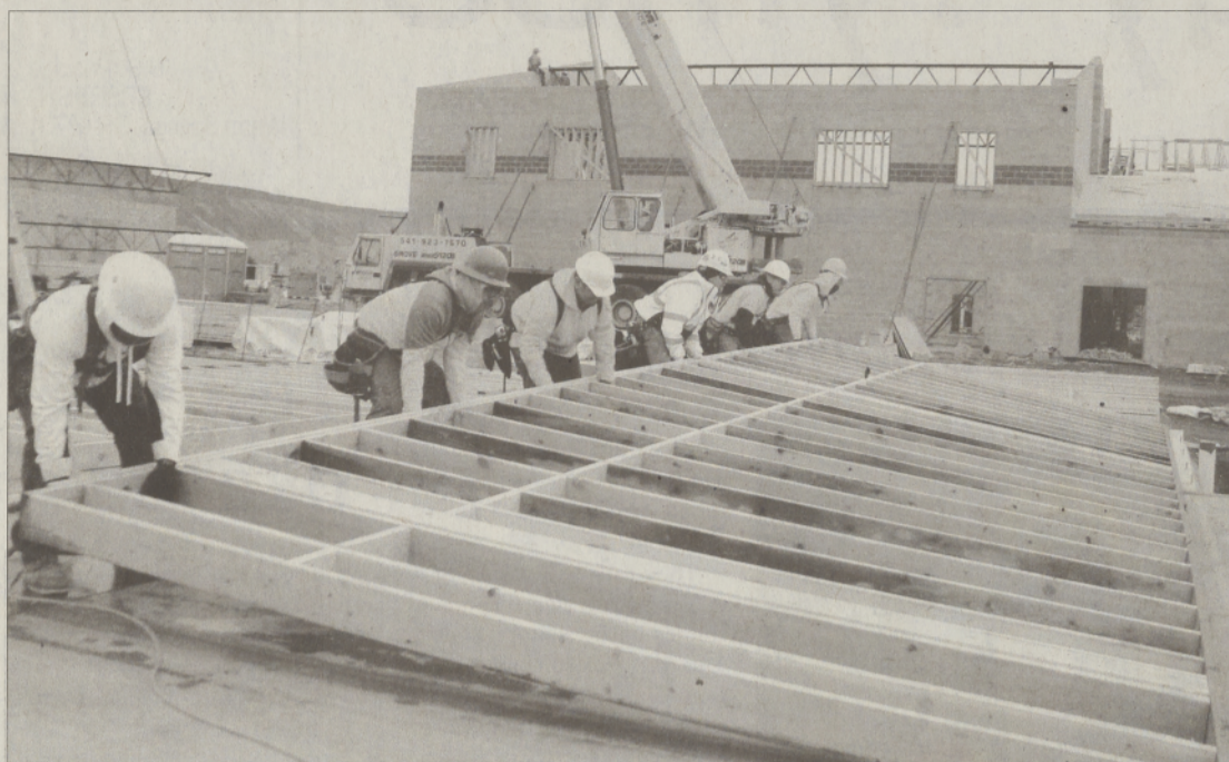
Workers raise a wall at the Warm Springs K-8 Academy.
