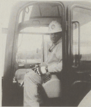
Casey Green of Warm Springs flashes a smile while working on Warm Springs K-8 school construction.
