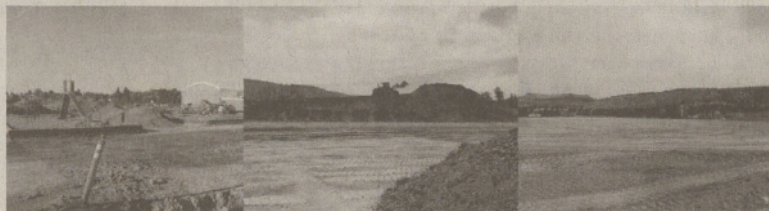
(Left) Madras Primary play yard and parking lot. (Middle/right) Warm Springs K-8 football field under construction.
