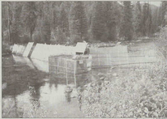
A weir across Johnson Creek allows tribal biologists to collect wild fish for broodstock while remaining fish are passed upstream to spawn.
