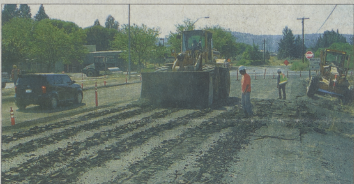
Construction crew at work on paving project.
