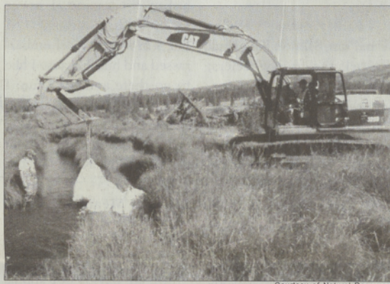
Restoration work during phase 1.
