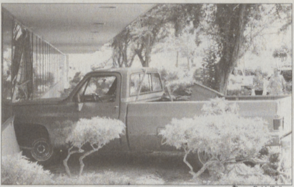
The truck hit the front of the admin building.
