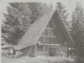
This is the building, Kirk Hanna owner of Mt. Hood Ski Bowl has offered to house information of the Confederated Tribes.
