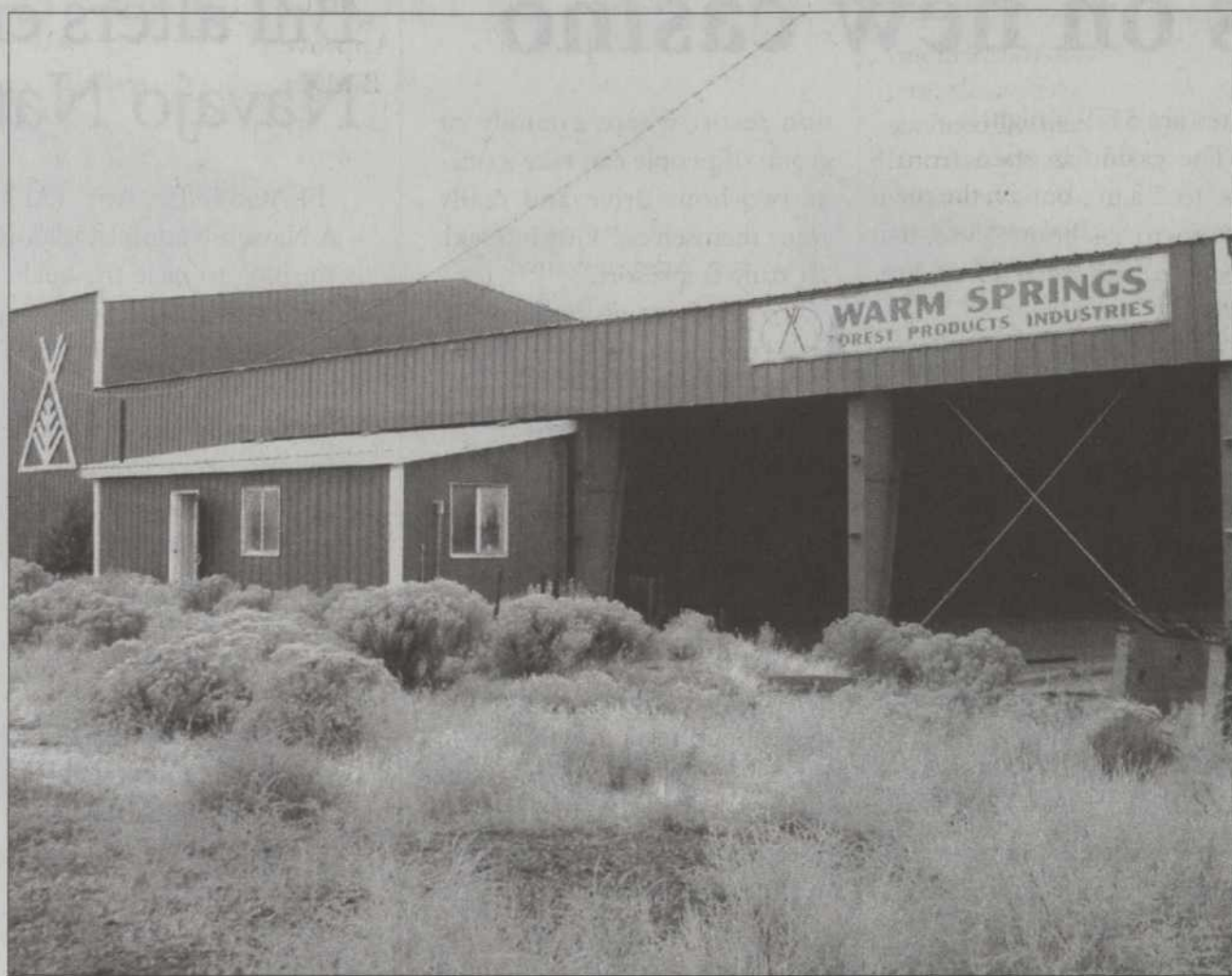
The development site is the tribal trust property at the Madras industrial park.
