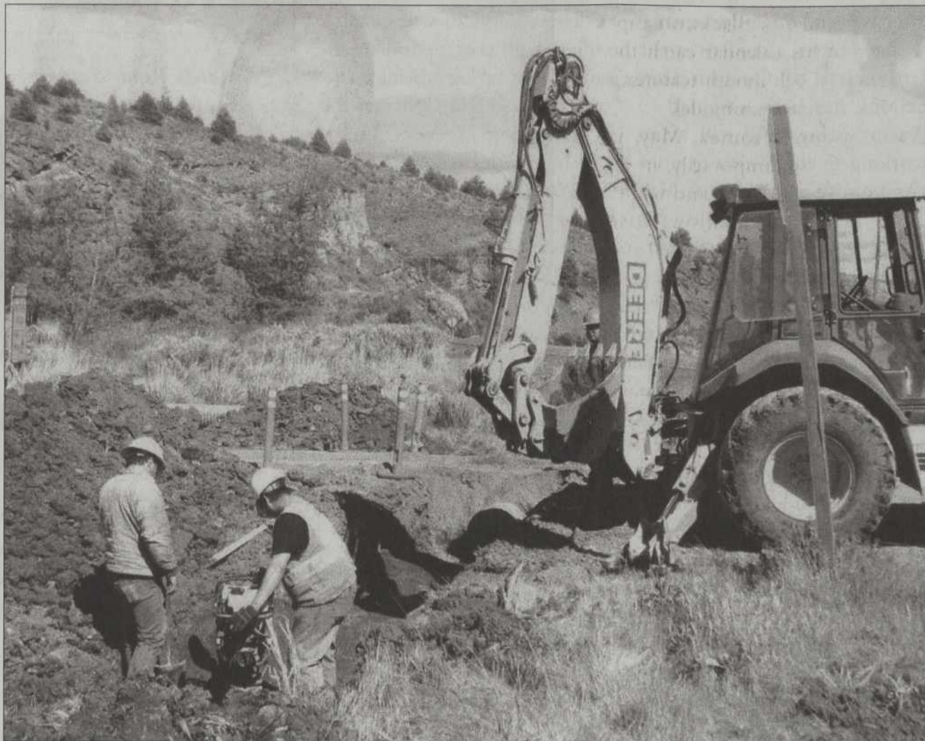
Lei Calica (right) and co-worker at Charley Canyon Project site.
