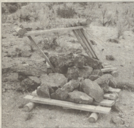
One project was to rebuild a rock fencing post. Below is the demolished post; and above, the rebuilt post.
