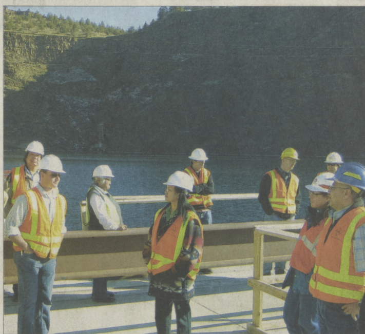
Tribal Council, management, PGE and Corps of Engineers officials last week toured the intake tower and fish passage facility that is under construction at the Round Butte dam.
