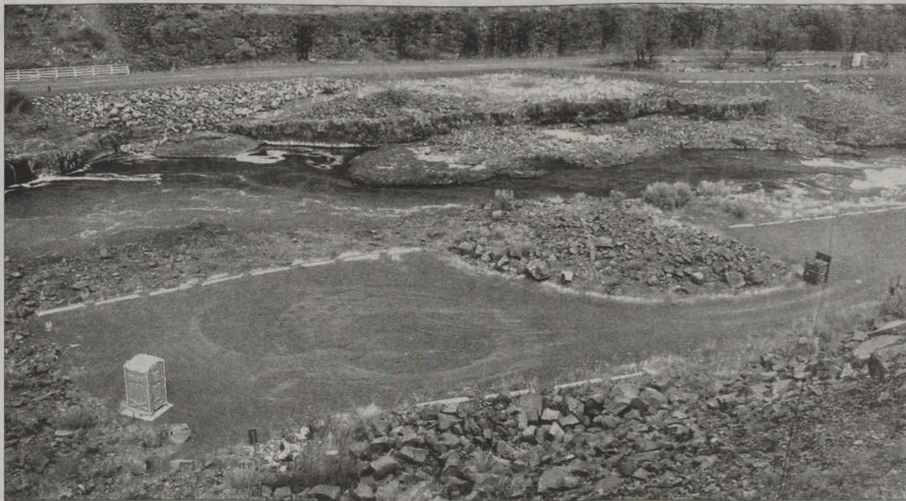
The parking area at Sherars Bridge was damaged.
