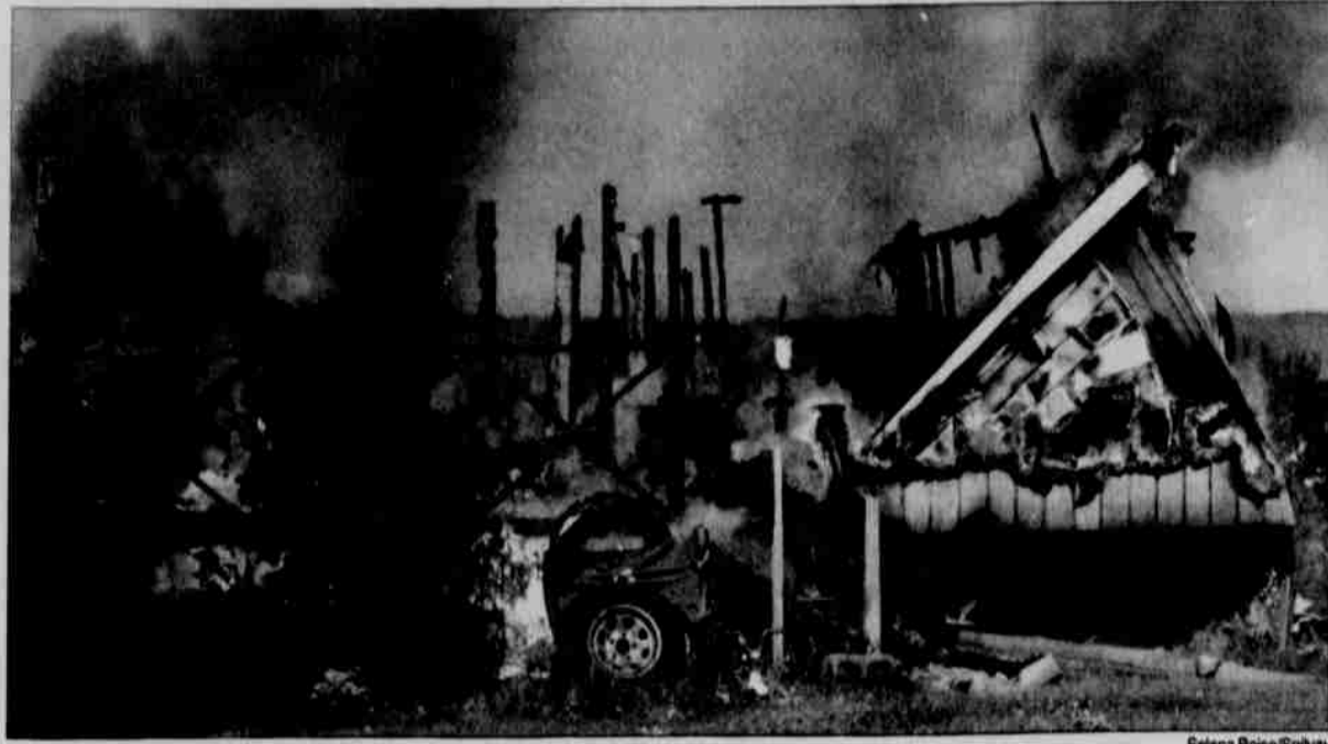
A few days after the house was destroyed by an electrical fire, the Fire Department cleared the property for safety by control-burning the remainder of the structure.
