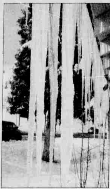
Icicles several feet in length formed at the WEDD building.
