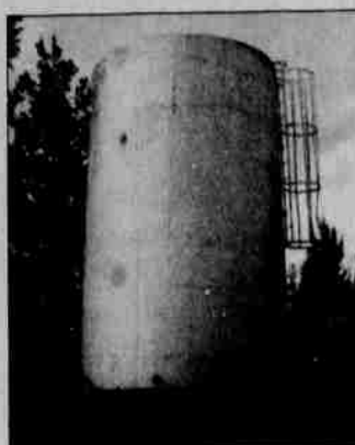
Near the new fire hall and residence is a water tank that holds 16,000 gallons; the water
