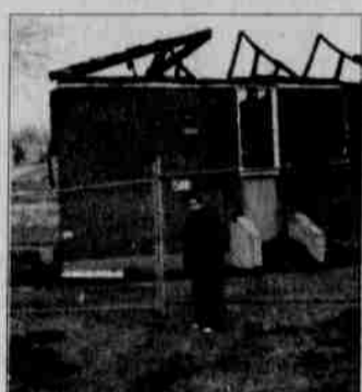
The gymnasium area was fenced off following the blaze.
