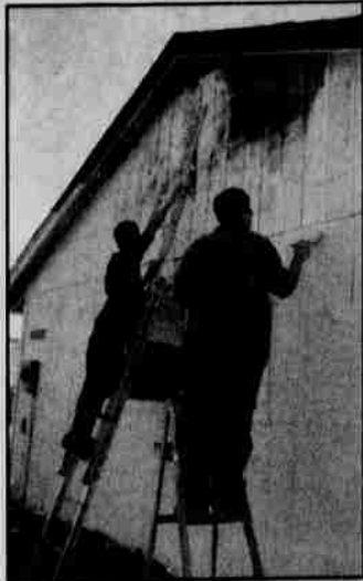
Two workers hard at painting.
