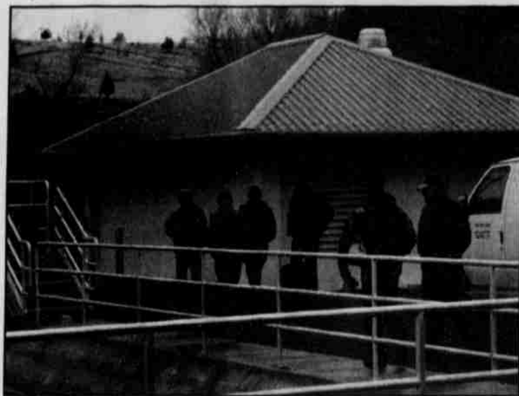
A group of inspectors from various government agencies, including those of the Confederated Tribes, inspected and then gave approval to the new Warm Springs Wastewater Treatment Plant, completed during the month of December.
