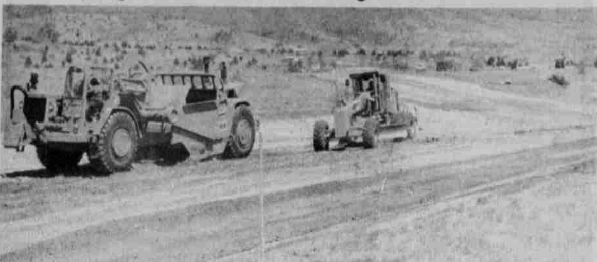
Heavy equipment at the new road construction work site.
