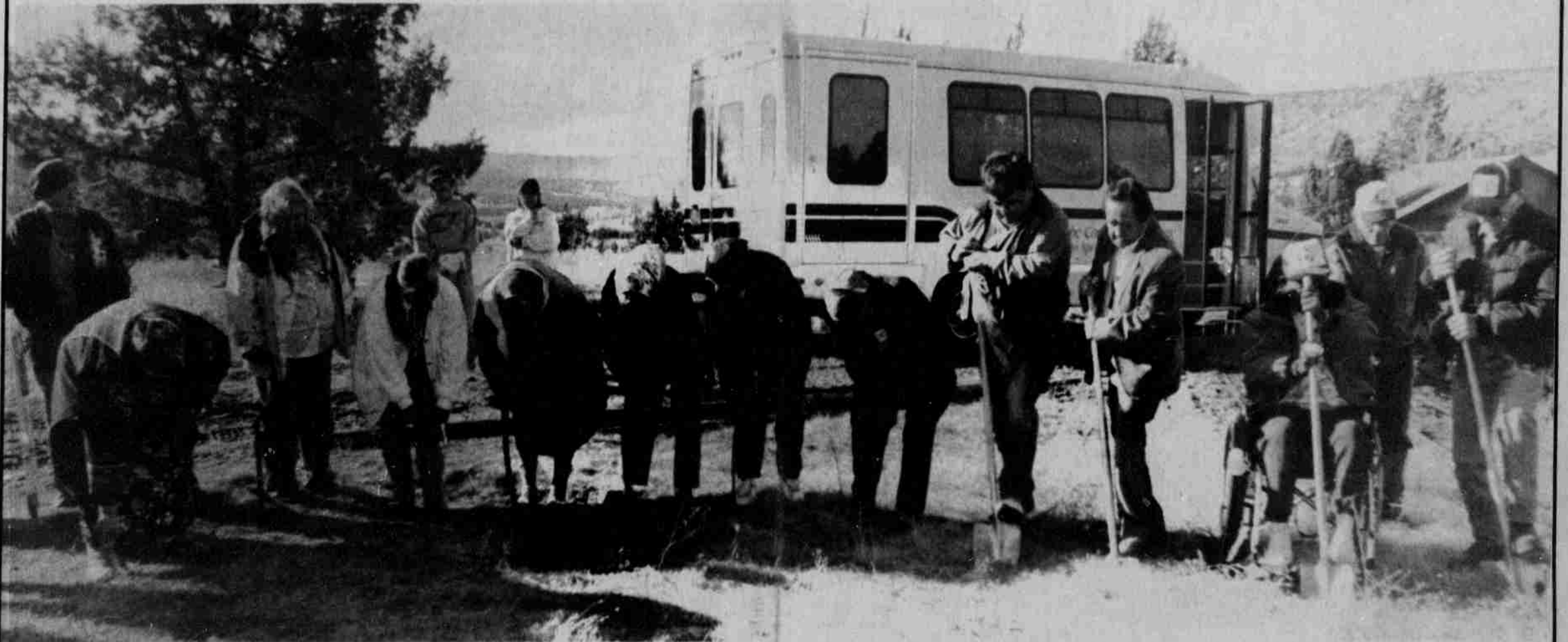
Groundbreaking was performed by Senior Citizens and dignitaries using shovels and kup'n's.
