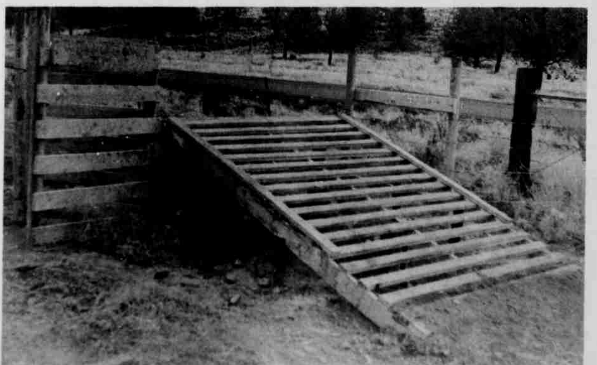
Ramps built for passing through without the need to open and close gates to pass through. Not recommended for taking jumps or passing over at high speed.
