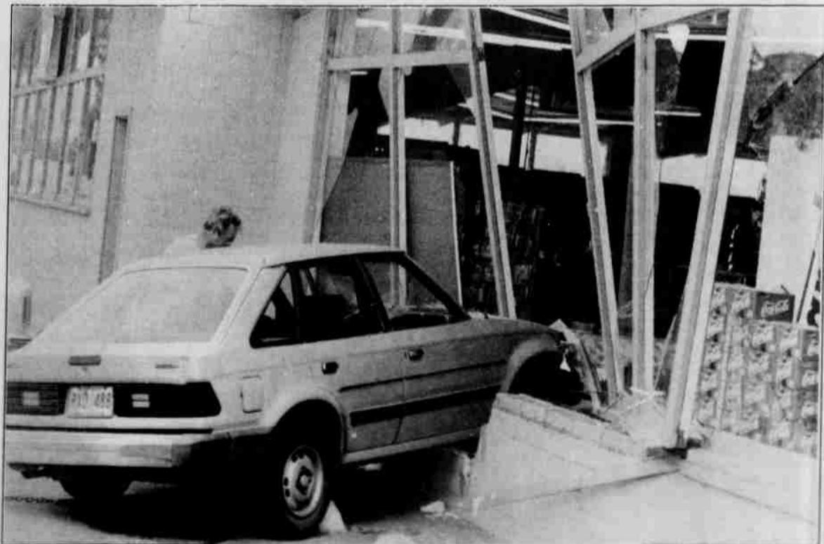
An unidentified driver tried to make Warm Springs Market a drive-thru Tuesday, June 17. No details of the accident were available, and fortunately, no one was injured. The store remained closed for the day until temporary walls could be erected and reopened June 18. The building will soon be remodeled.
