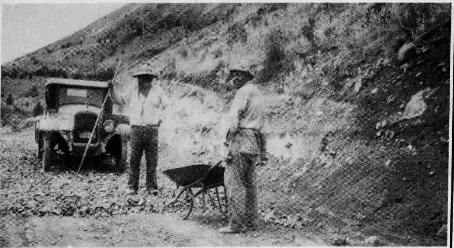
Warm Springs Reservation Indians at work on road from the Agency to Mecca, 1928. Photos by Pat Gray.
