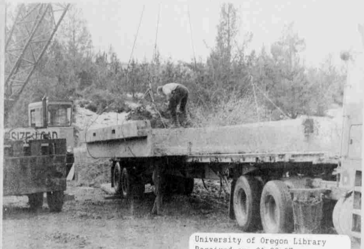
Pieces of the Thompson bridge were brought by trailer.
