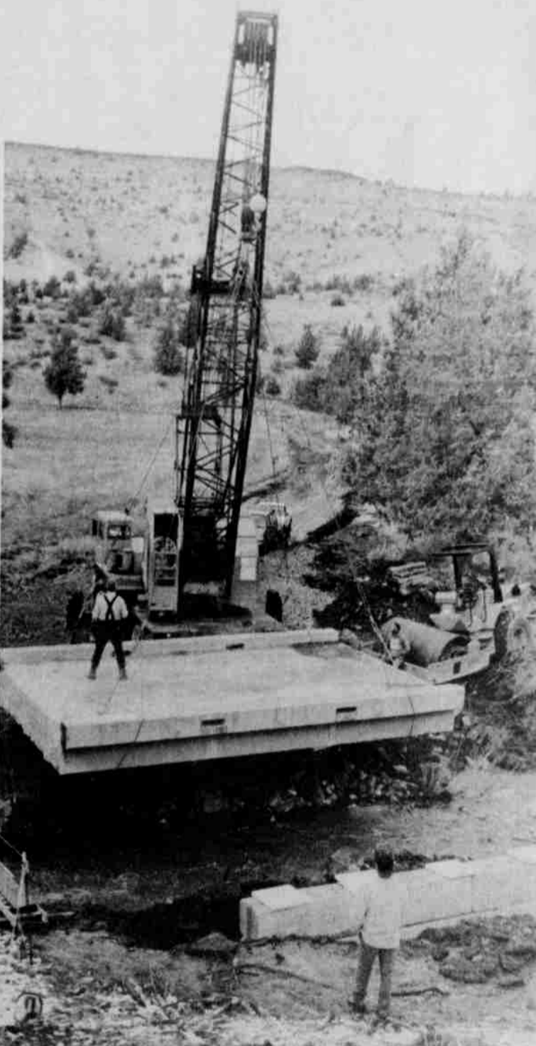
A piece of Thompson bridge was placed on Palmer Drive where flood overflowed culvert.
