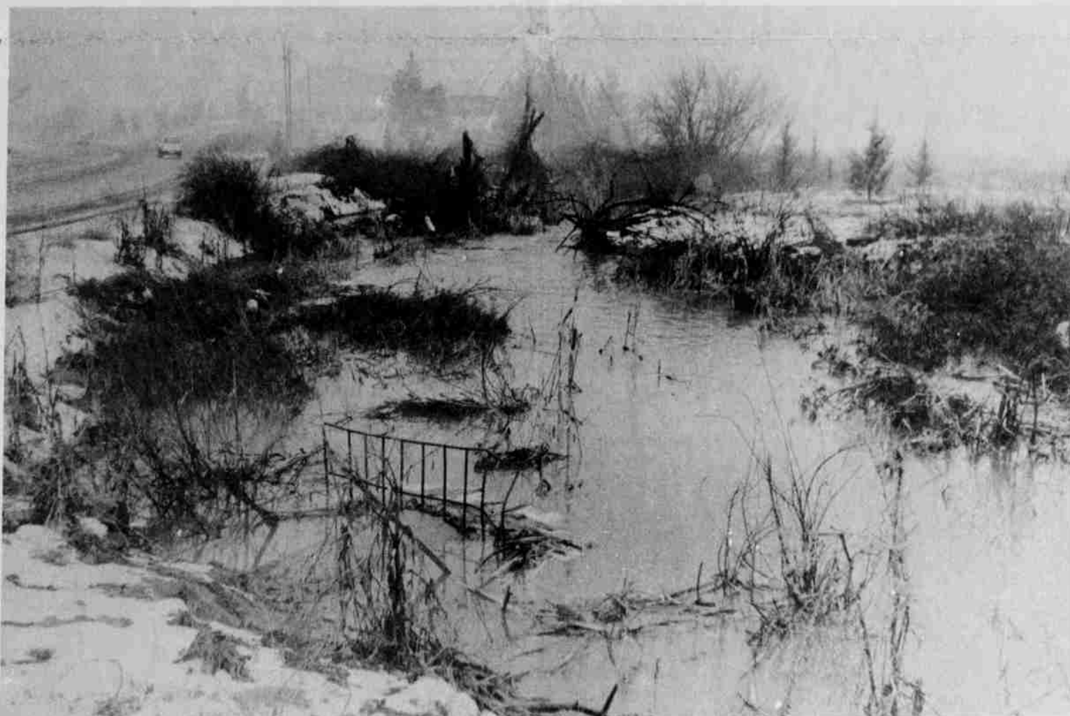
Drainage pipe along intersection of Tennino and Hollywood clogged up with debris sometimes causing water to collect
