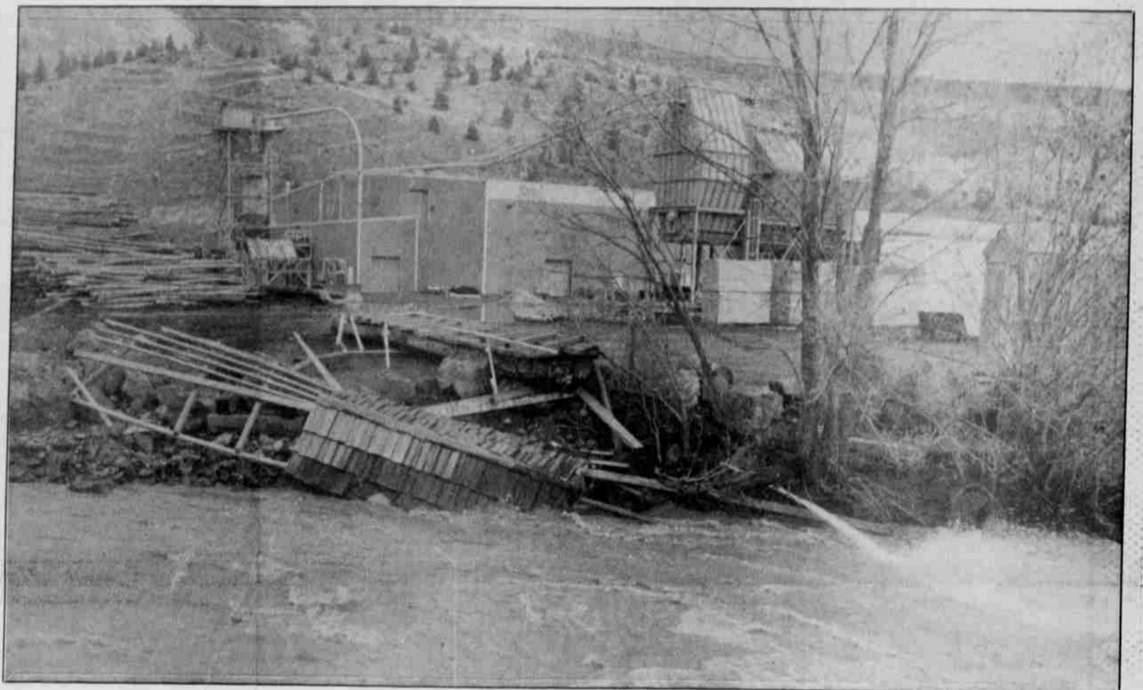
The footbridge joining the mill yard and office was washed away during the high water.
