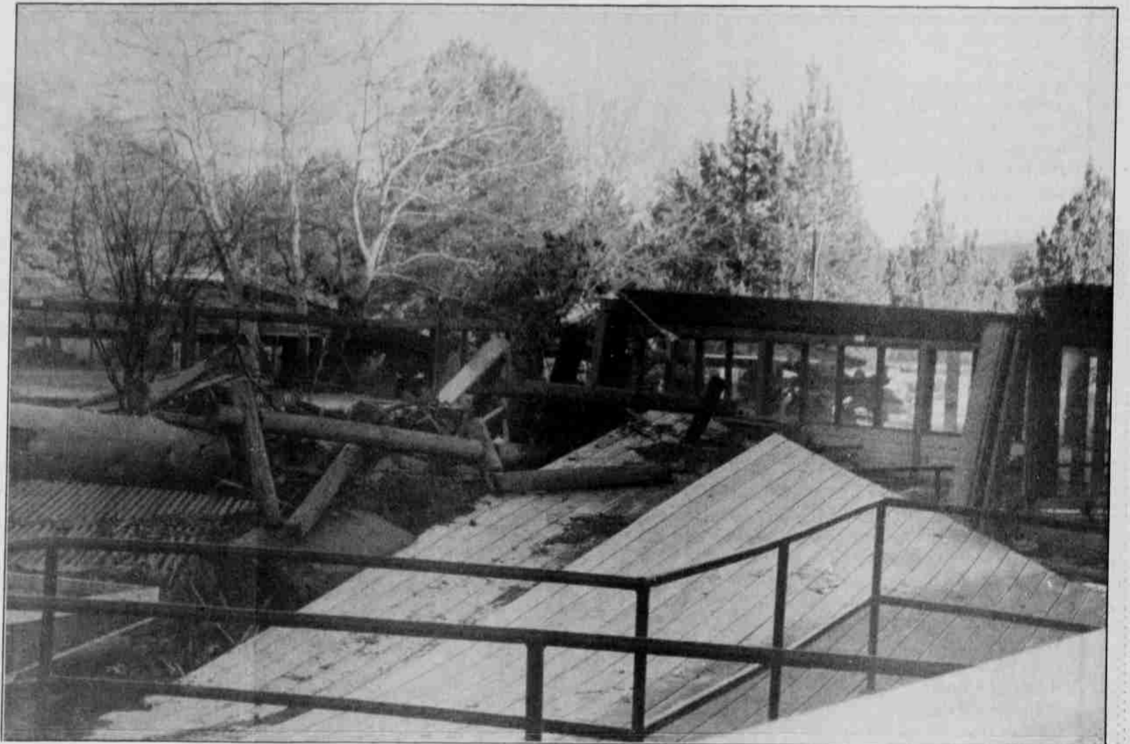
Village pool decking was tossed around by the powerful current.
