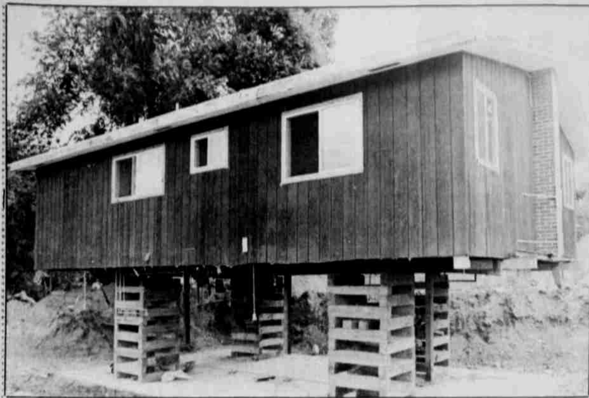
Nina Rowe's house in Elliott Heights has been lifted off its foundation so that complete remodeling can take place. Another house across the street is undergoing the same treatment.
