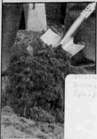
Earth was turned for official beginning of construction.
