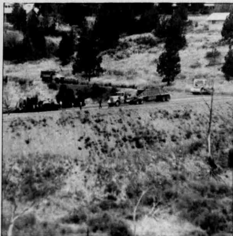
Construction work on change of North Hollywood Street.
