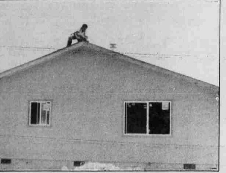
Private contractor Tom Kalama finishes roof on recently constructed Sunnyside home.
