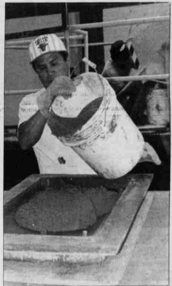
Frank Smith pours slurry into form.
