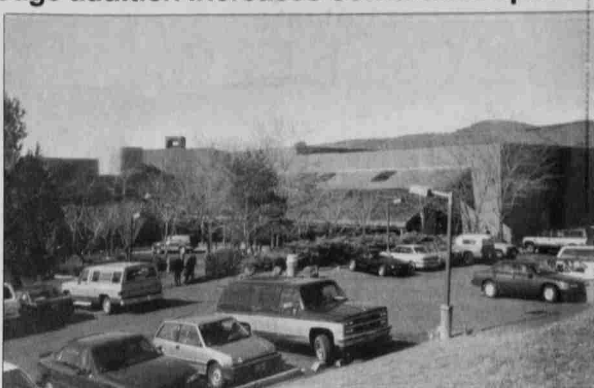
An addition on the north side of Kah-Nee-Ta lodge allows easy access as a meeting room and provides needed conference space.
