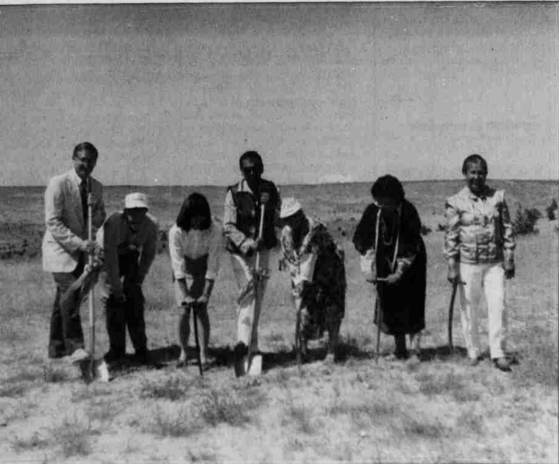
HUD executive director Jerry Leslie, future home owner Randy Thomas, architect Leslie Harashick, and Local Housing Authority members Elton Greeley, Lizzie Rhoan, Neda Wesley and Arlita Rhoan broke ground in the Sunnyside Subdivision recently, marking the start of construction of 30 demo project homes. Construction is due to begin by the middle of this month and be completed by April 1993.
