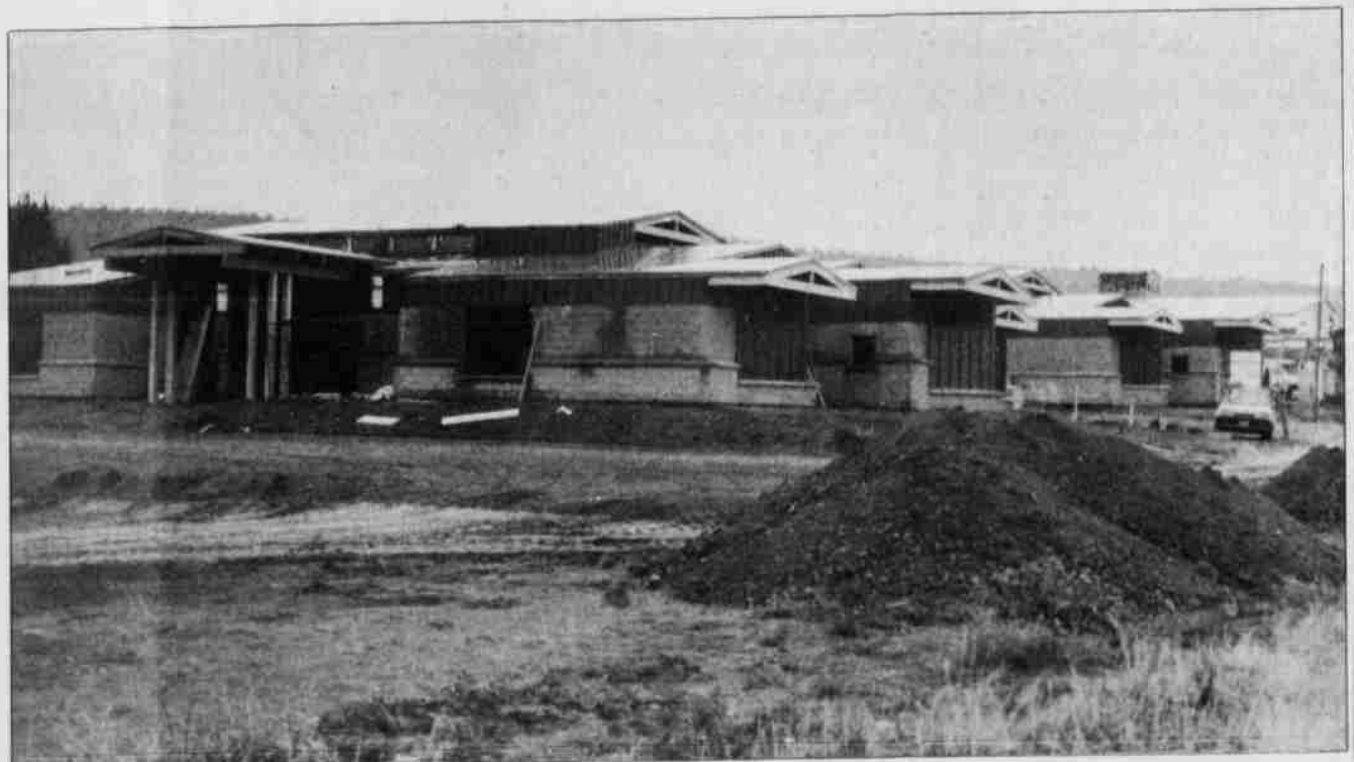
Early Childhood Development Center is expected to be completed mid-year 1992.
