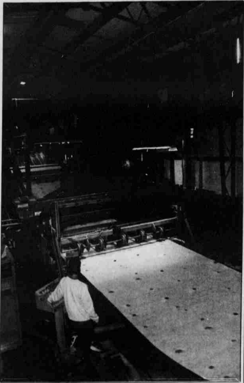
The veneer plant has undergone considerable renovation over the last three years. The laser controlled clipper was installed in 1988 and a cold charger scanner was installed earlier this year.
