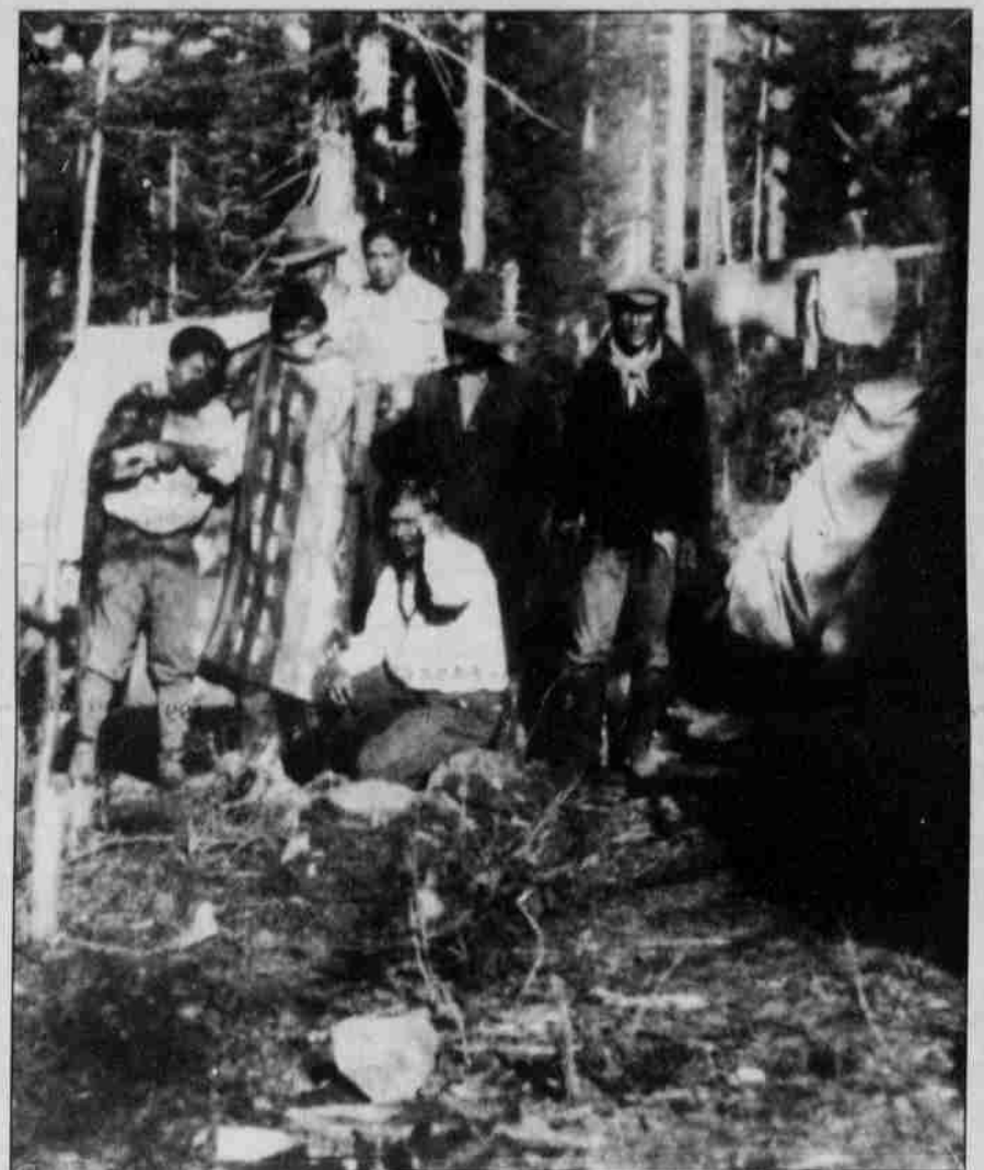
Home for loggers were tents in the forest
