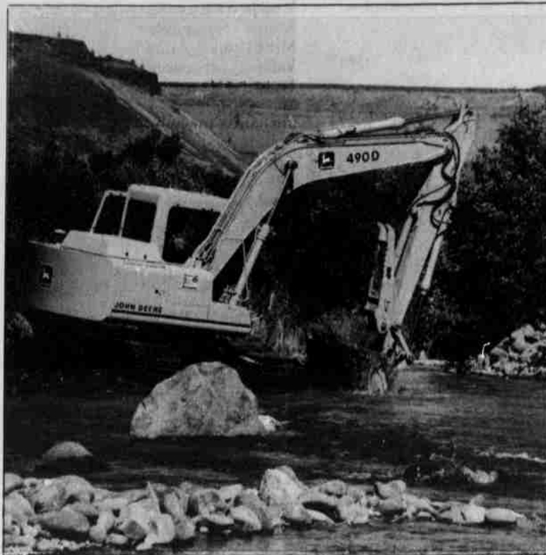
Integrity of Shitike Creek is protected during museum land stabilization work. Boulders provide rip-rap and prevent fill dirt from washing away.
