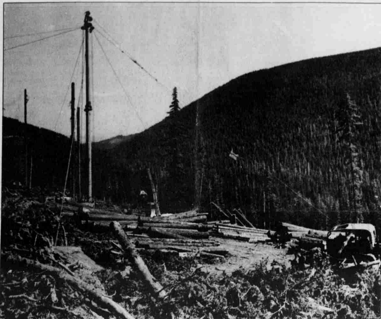
Timber off the Vantage sale unit is being exported to Japan. Part of the unit is logged with high-lead cable.
