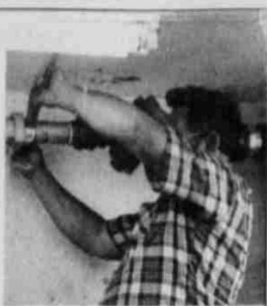
Water and wastewater foreman Ron Maitland repairs broken water valve.
