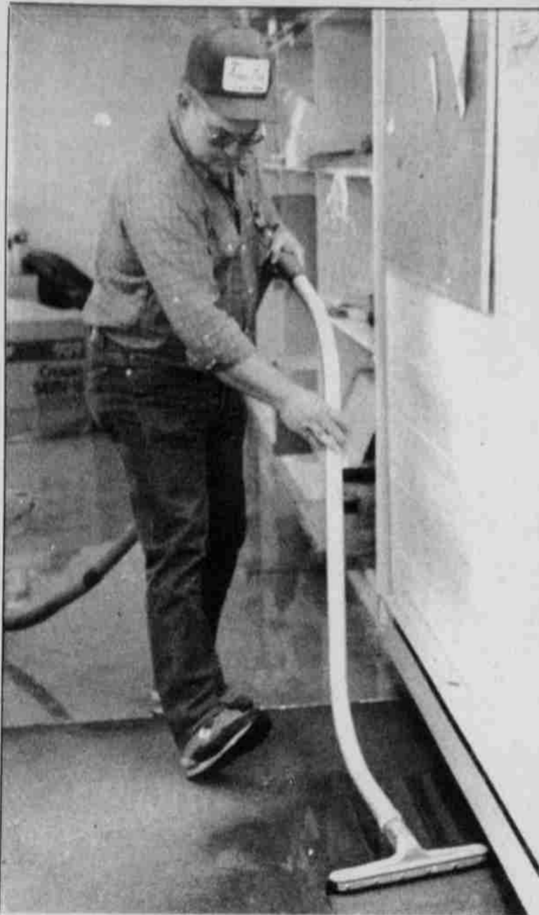
Tribal plumber Cliff Stallings helps vacuum water that covered the floor of Spilyay Tymoo offices.
