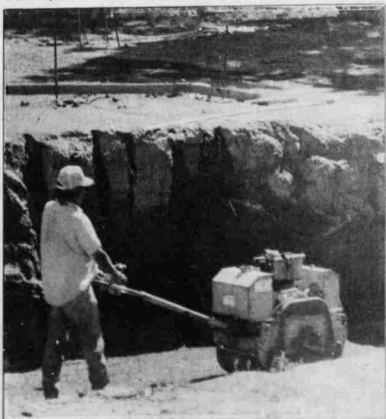
Construction worker prepares the ground for new office foundation.
