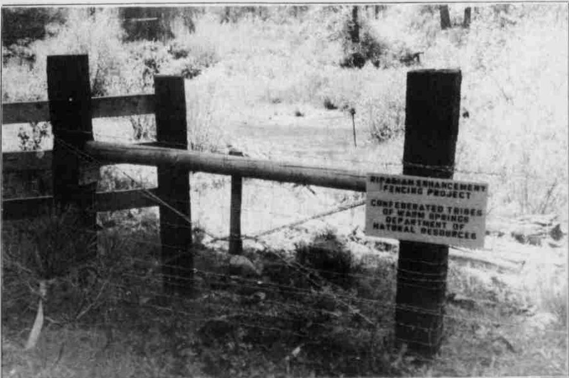
A recent fencing project on Beaver Creek will help protect sensitive streamside areas from livestock which tend to compact the soil and denude areas of vegetation. This is one of many projects on the reservation designed to protect water quality and quantity.
