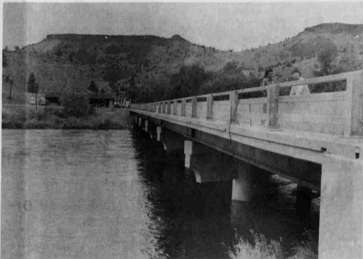
The newly completed bridge is nearly double in size and makes for safer travel.
