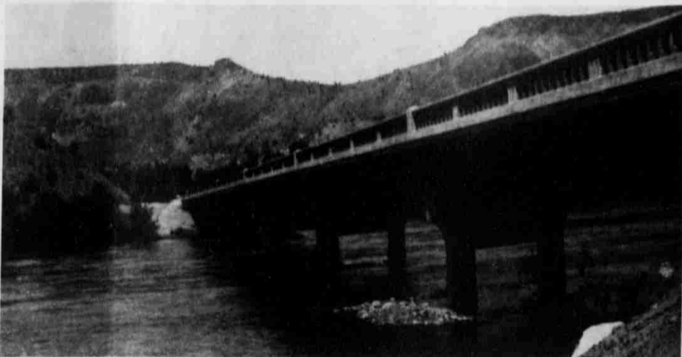
The original Deschutes River bridge was built in 1934.
