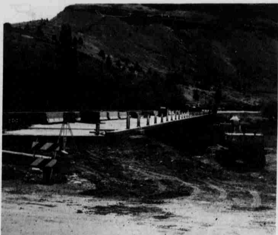
Construction on the bridge ran from June 1987 to November 1988.
