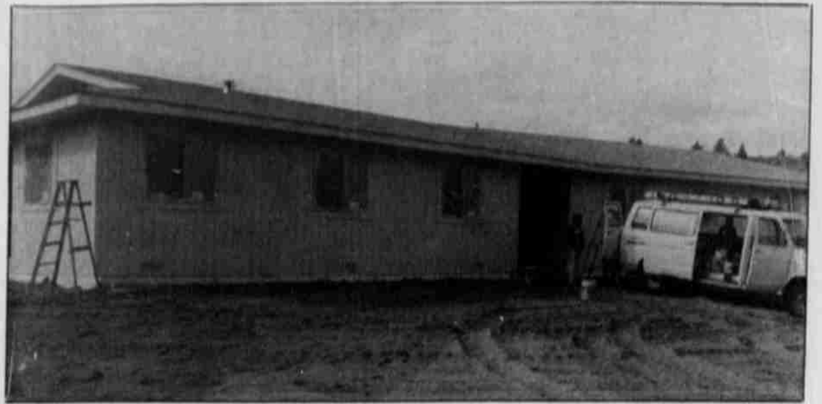
Foresters relocate Two new buildings located at the Fire Control complex in the Warm Springs Industrial park will allow Bureau of Indian Affairs Forestry department personnel to move from the basement of the old administration building. The new buildings will be occupied in October.
