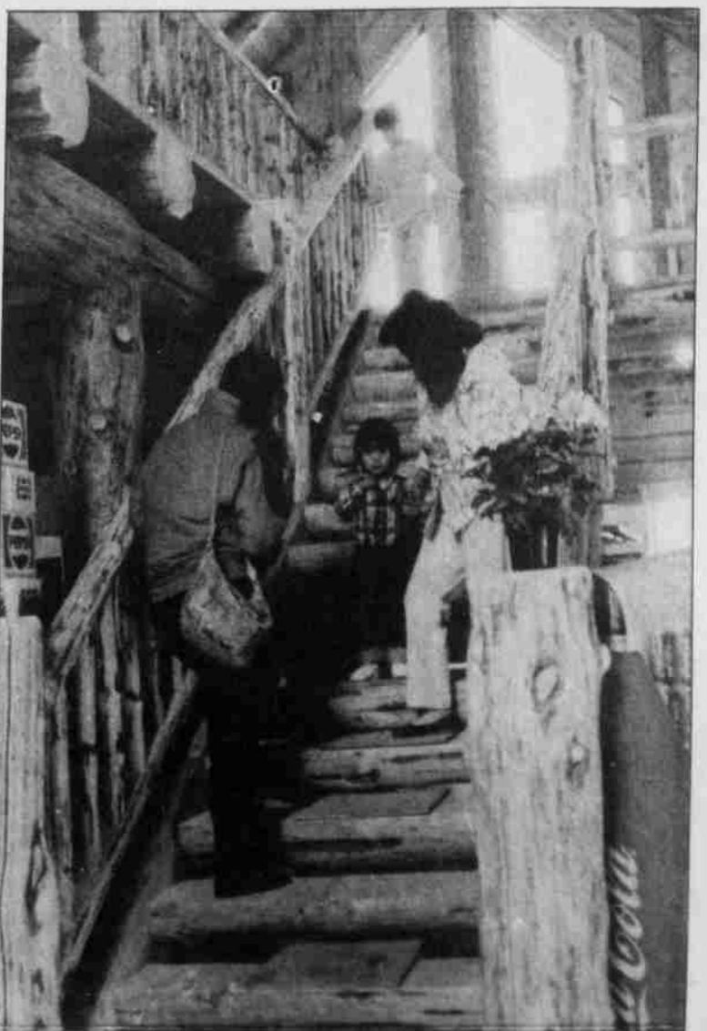
The grand opening of the new Charley's Market went off as scheduled Saturday, March 21 although the market's inventory consisted of only pop and gas. Work on the log structure is continuing with touches of detail work. Frank Charley stated that actually it will probably be about four weeks before the store will begin selling with a fully stocked inventory. He estimated that in the neighborhood of 900 people attended the opening and the traditional meal served in the longhouse commemorating Simnasho's first store. Many young people attending the opening were not hampered by the lack of inventory in the store, they were busy taking turns trying for the highest score on a video game in the store.
